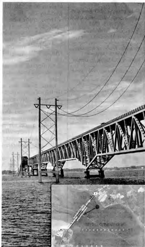
This rendering, furnished by Dominion Virginia Power, shows a simulated view of the new towers and transmission lines parallel to the Robert O. Norris Jr. Memorial Bridge. The red indicator (inset) shows the perspective for the larger image.
